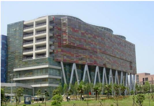
**Inotera Fabs 1&2** (Taoyuan, Taiwan): Structural and mechanical vibration design of two 300mm DRAM (memory chip) factories. For both projects, we proposed a moment frame system with no interior shearwalls and unified structures. We utilized small shearwalls at the perimeter of the manufacturing floor to carry lateral loads. This design enhanced subfab space management and is an accomplishment for a tall structure with micro-vibration requirements.
